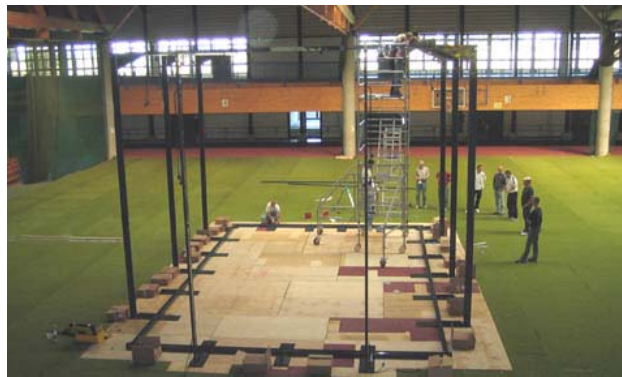
A glass court under construction in Europe
